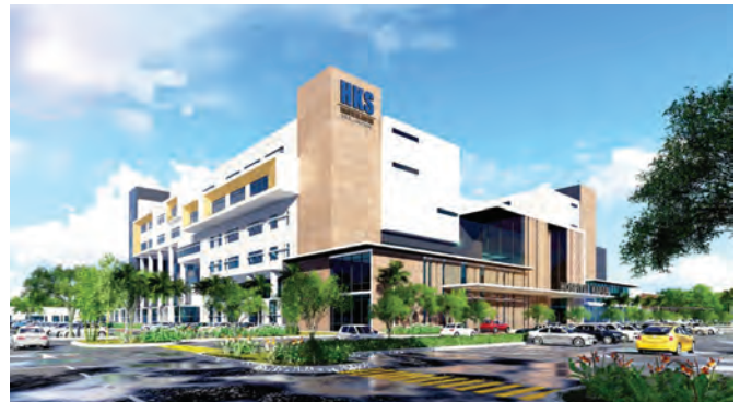
The construction of Hospital Kapar in Selangor, Malaysia, is scheduled to complete by November 2026.
