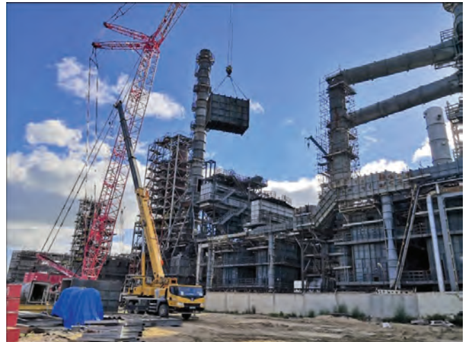
Using MyCrane's online crane rental platform, Beijing-based Haihua sourced a 400 t crawler crane for use on three column installations at a refinery.
