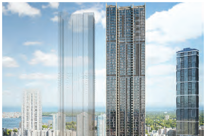
Construction work on the project involves the delivery of a 70-storey and a 72-storey residential building.
