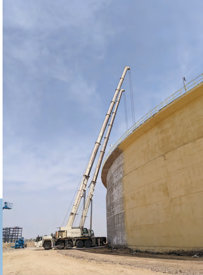
OPPOSITE, ABOVE AND BELOW: Steel Carriers used eight Tadano all-terrain cranes to lift a 250-t dome with a diameter of 126 m evenly to a height of 16 m.
